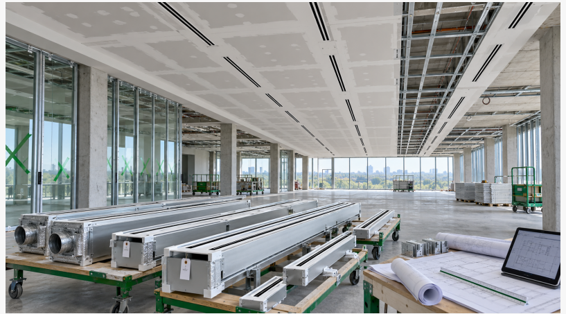
Linear diffusers and HVAC components staged in a commercial interior during drywall finishing. Not an actual Cryptic Air project.
