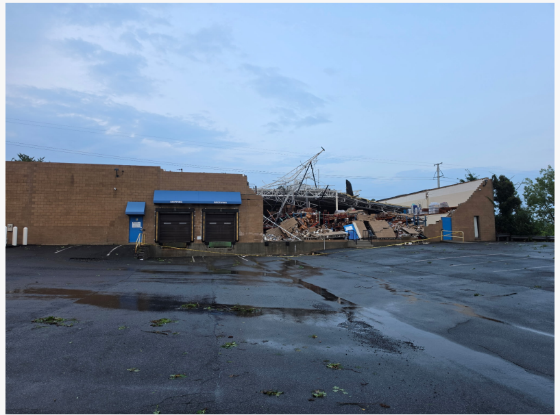
Bead Electronics' manufacturing facility immediately following the storm, which caused extensive roof, warehouse and water damage and temporarily halted production.
