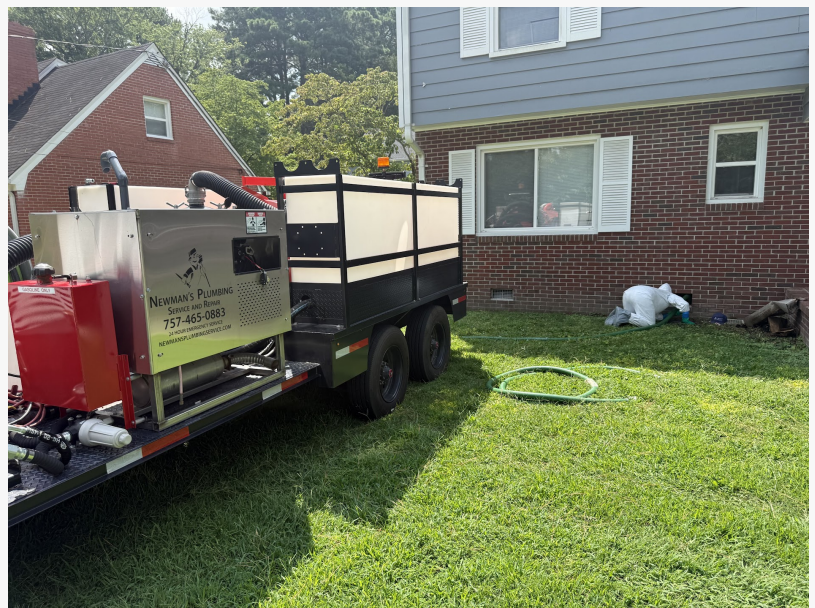
Newman's Plumbing technicians use HydroVac excavation equipment for utility-safe digging.
