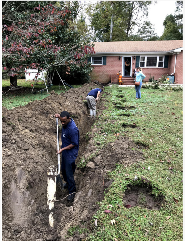
Newman's Plumbing technicians excavate a trench for a water or sewer line repair.
