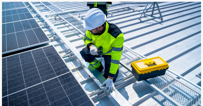
Solar Commercial Contractor on Roof
