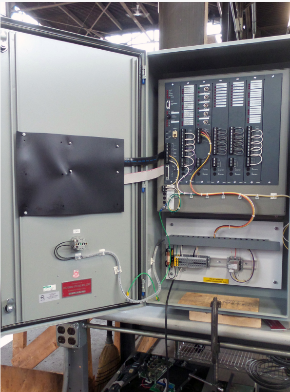
Fuel System Controller for a data center.
