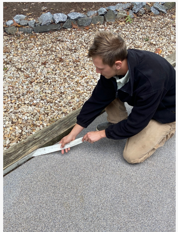
Final steps of removing tape from wood surrounding Terrazzo patio application.
