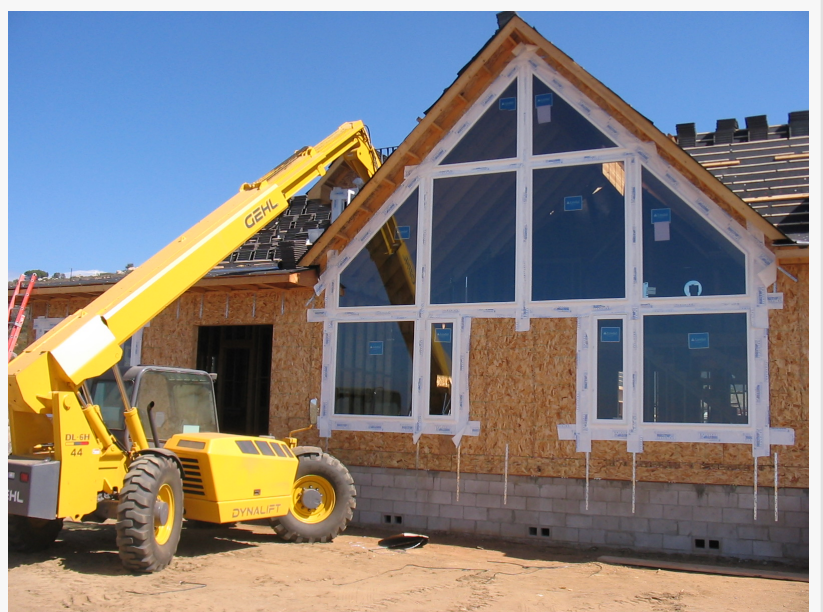
Window Solutions New Construction Window Installation
