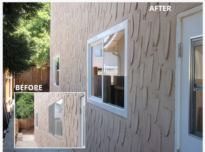
Window Installation in Lakeside
