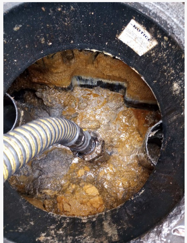
Professional grease trap cleaning underway to remove accumulated FOG and restore proper operation.
