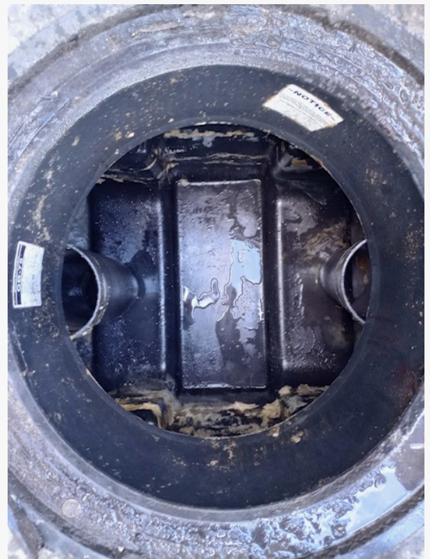
Clean grease trap after professional pumping at a Los Angeles restaurant
