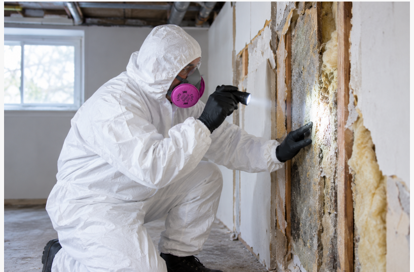
A certified asbestos inspector examines exposed wall cavity insulation during a pre-renovation survey.
