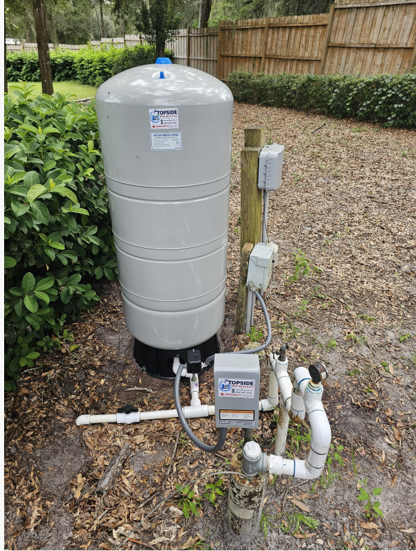
Emergency Well Tank Replacement Ocala Florida
