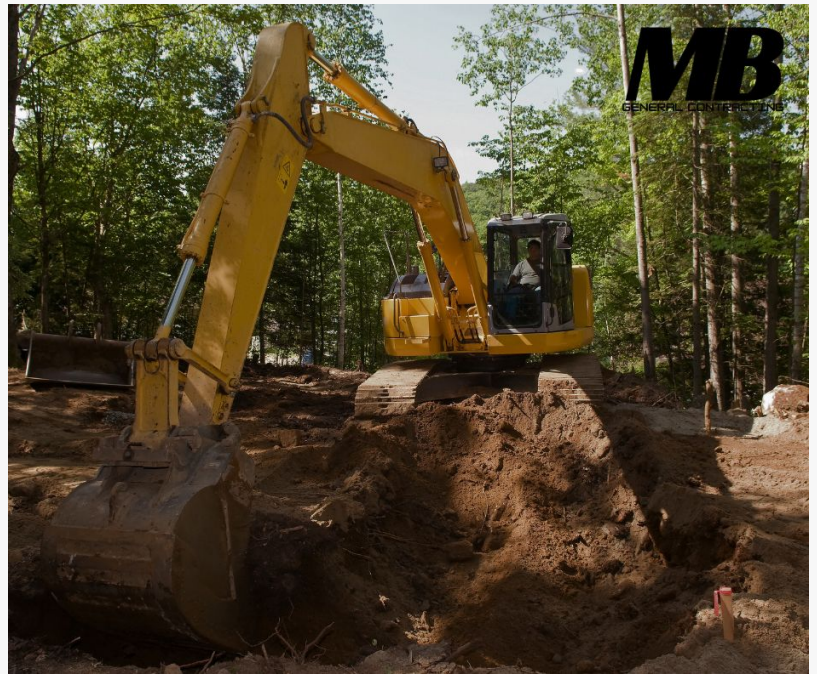
Site Preparation Services in St James MO
