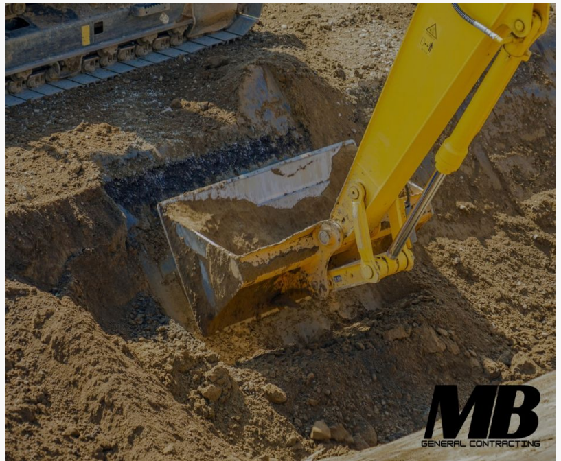
Recent Commercial Excavation project in the St James MO area
