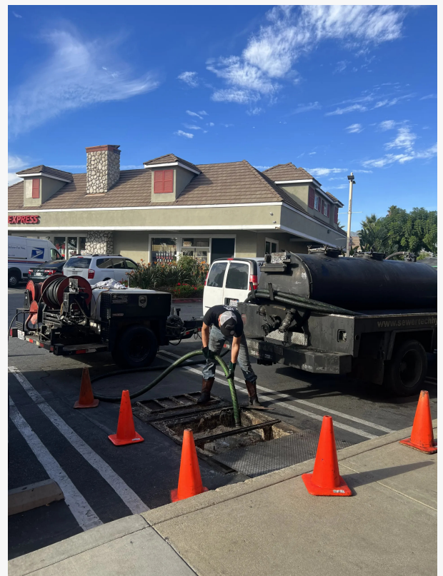
The Grease Company technicians pumping an underground grease interceptor at a commercial property in Southern California
