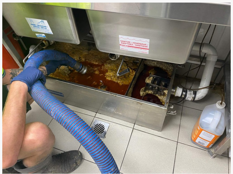
Professional grease trap pumping service in a commercial kitchen in Los Angeles County
