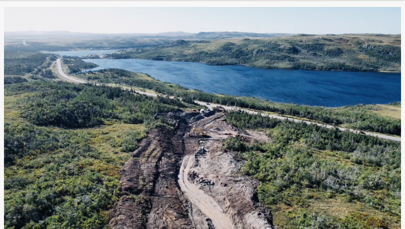
Entrance to SLC-01 of the Atlantic Spaceport Complex (ASX) Under Construction
