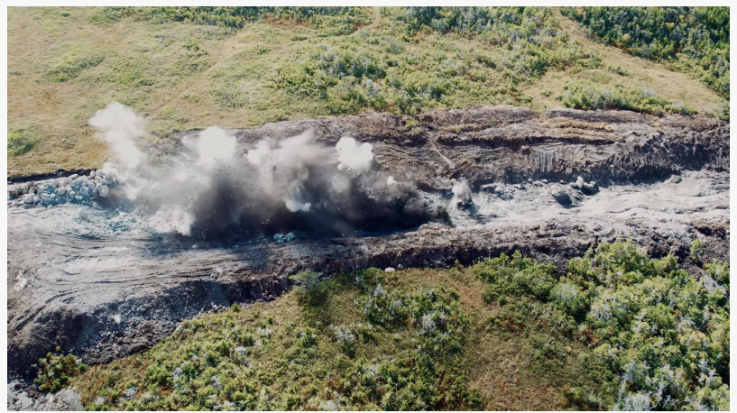
Frequent Blasts Ongoing at the Atlantic Spaceport Complex (ASX) SLC-01
