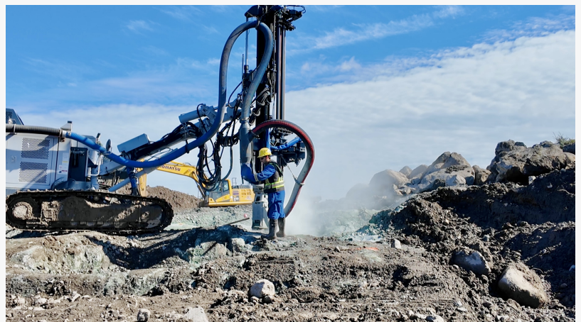
Construction In Progress During Phase 2 for SLC-01 at the Atlantic Spaceport Complex
