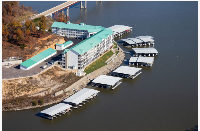
Client-provided aerial view of waterfront docks at Lake of the Ozarks. Atlas Docks serves residential, commercial and shared waterfront structures.
