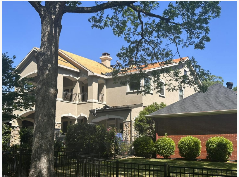
A J. Cole Roofing and Construction crew member works on new roof decking during a residential roof replacement in Cabot, Arkansas.
