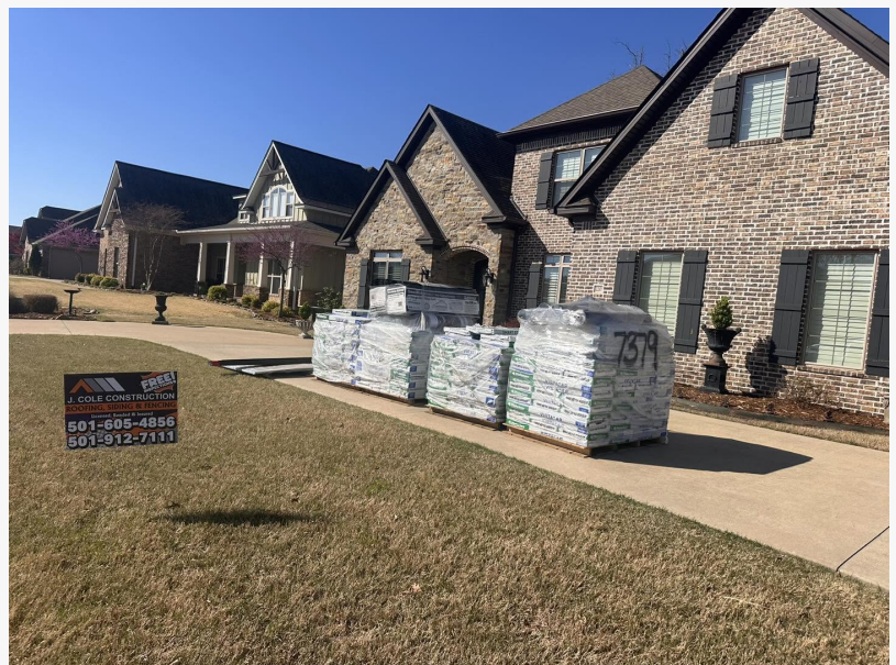
Shingle bundles and roofing materials staged at a Cabot, Arkansas home ahead of a J. Cole Roofing and Construction roof replacement.
