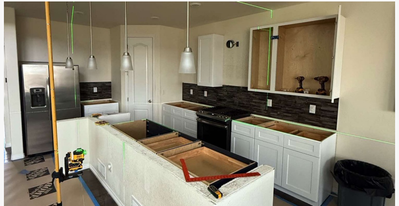
A kitchen remodel in progress by Elite Property Innovations, with new cabinets installed and a laser level marking layout lines for the island.
