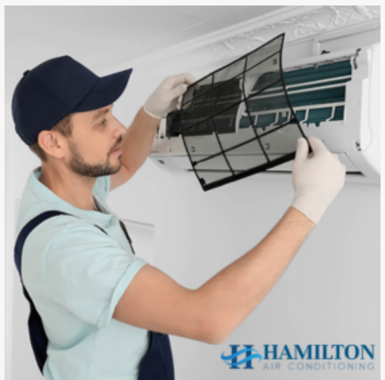
Reliable air conditioning services for homes and businesses
